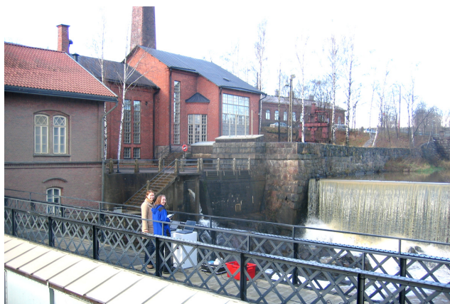
Fig. 1. The Vanhankaupunginlahti barrage with two happy measurers. The AIS took measurements from the bridge. The reference measurement point was about 100 m to the right (East) of the bridge. The closest road is located behind the building in the middle of the picture.
